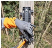
Fix the support plate using a minimum of two nails bonding with galvanised washer in the slots provided.
