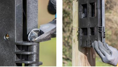
**2** Detach two fixing pins from the additional enclosure support.
