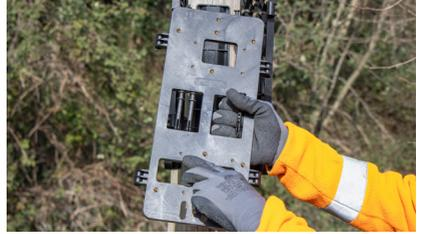
**3** Insert the third enclosure support. Secure it with 4 fixing pins.
