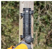
Fix the support plate using a minimum of two screws in the slots provided.
